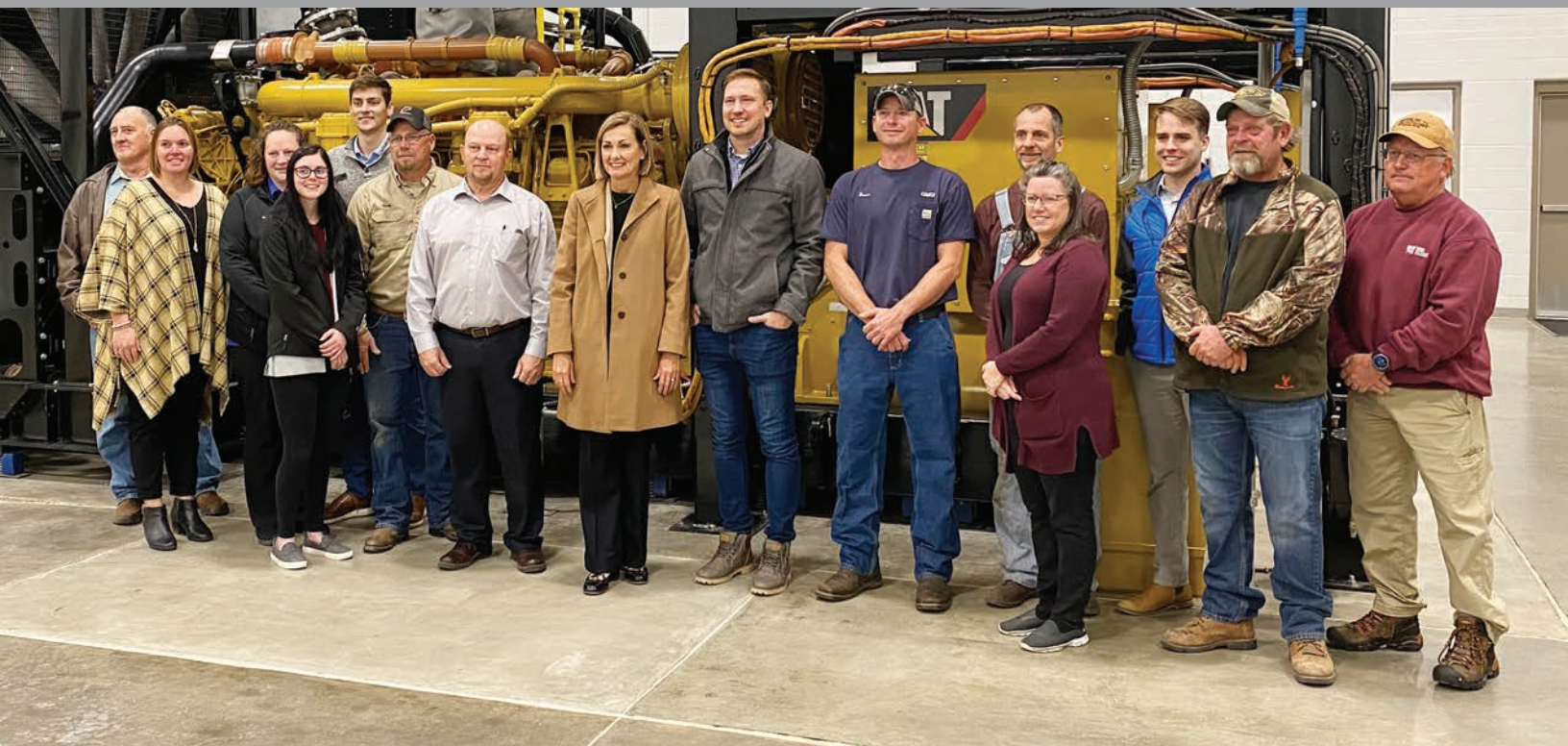
Iowa Governor Kim Reynolds and Representative Ray Sorensen, center, visit Greenfield Municipal Utilities' new generation plant in October, 2021.
