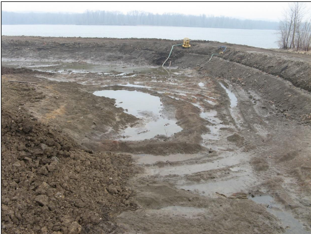
Photograph 4 | Dewatering during backfilling of the South Ash Pond, looking south. The water was removed to ensure placement and compaction of the backfill. | April 7, 2015
