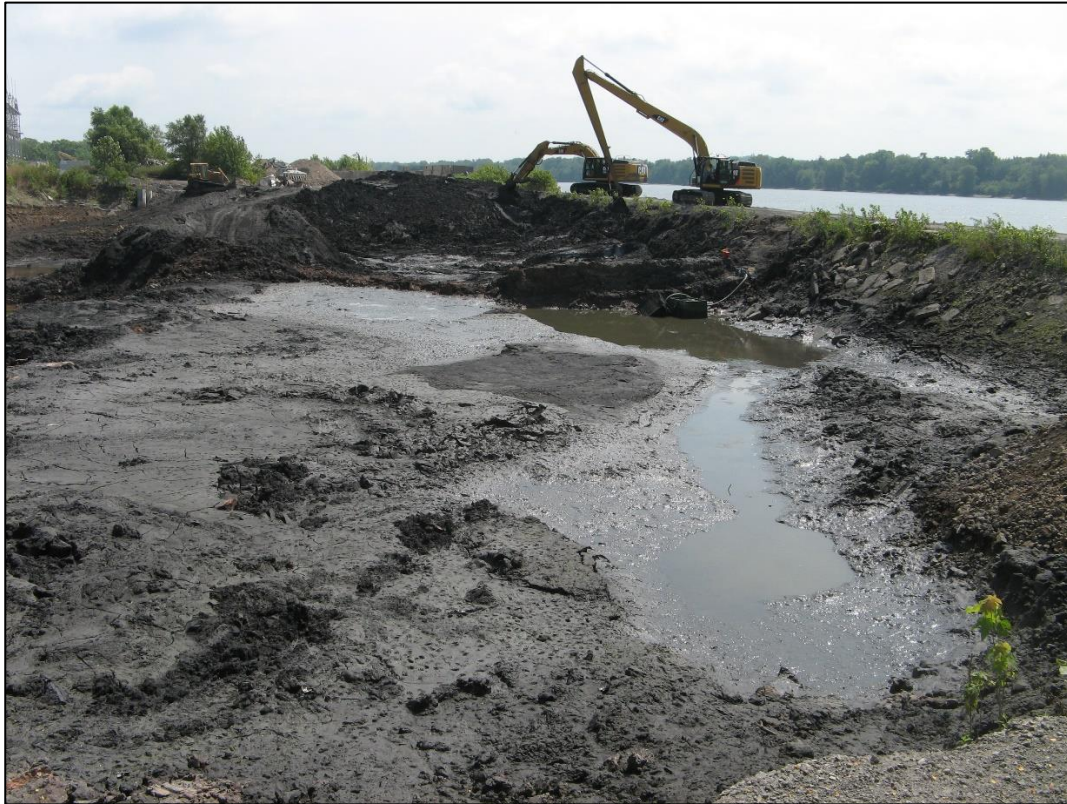
Photograph 1 | South Ash Pond during excavation, looking southeast. The dark material is CCR. | August 19, 2014
