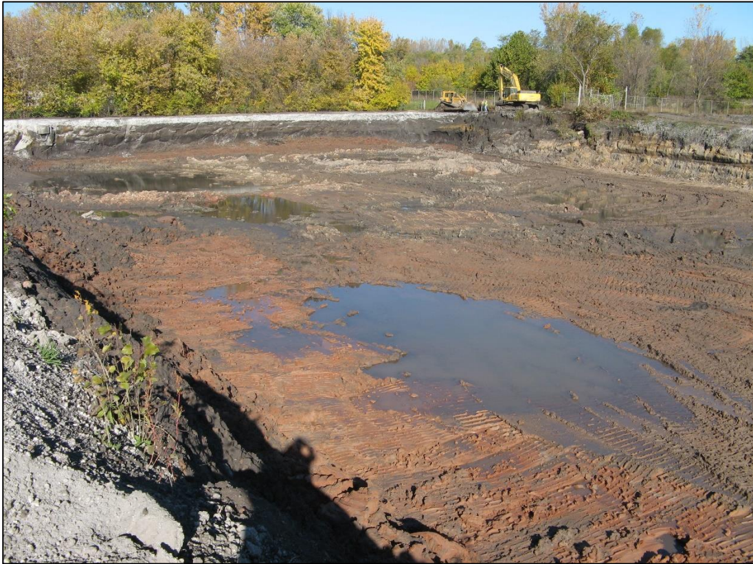
Photograph 3 | South Ash Pond after excavation was complete. Native soils in dark brown to light brown observed around perimeter and the floor. Viewed looking northwest. | October 22, 2014
