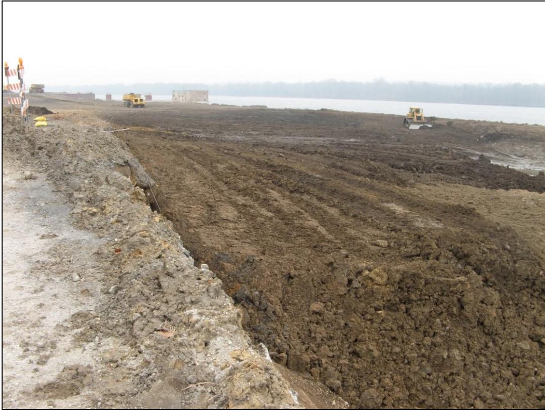
Photograph 5 | Backfilling of the South Ash Pond, looking east-southeast. View is to the east of Photograph 4 location. | April 7, 2015
