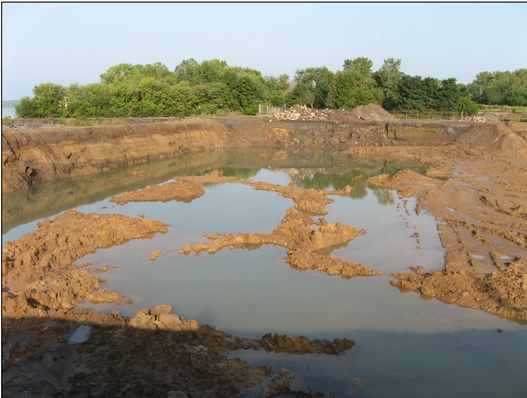
Photograph 2 | North Ash Pond with stormwater after majority of CCR removed. Native brown soils are observed around the perimeter and floor. View is looking west. | August 29, 2014
